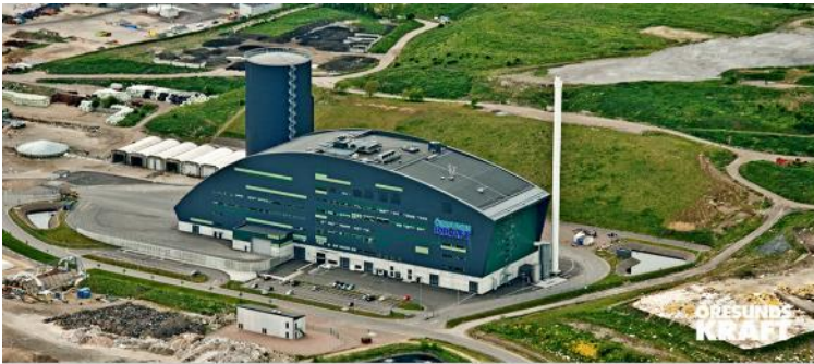
Figure 4 Filborna EfW plant
